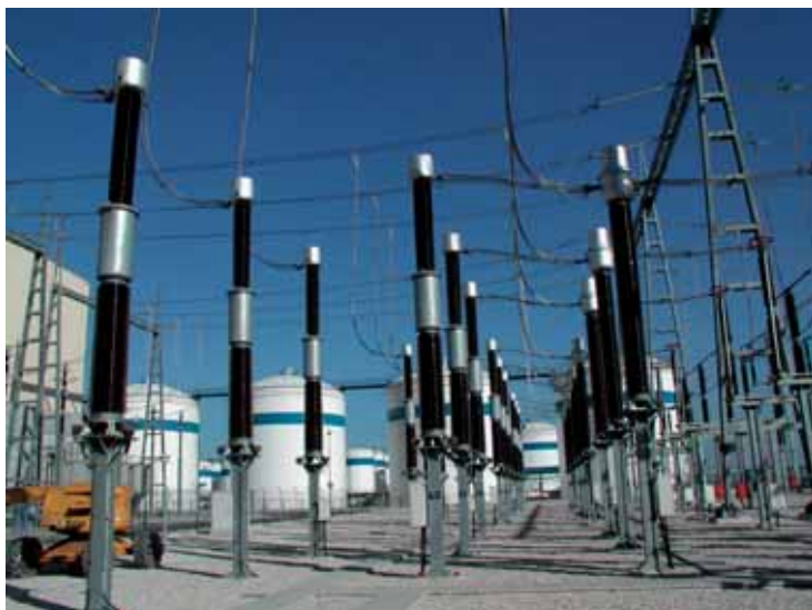
123 kV Inductive Voltage Transformers. Electronet Services (New Zealand).
