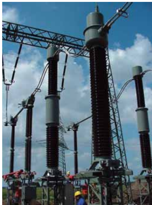
420 kV Current and Inductive Voltage Transformers. Vattenfall Transmission (Germany).
